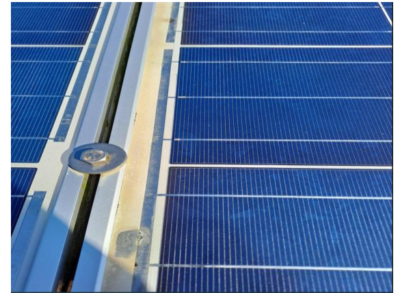
Example of bus-bar corrosion on a PV module
